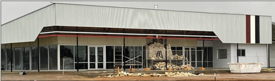
The new Western United Saints clubrooms under construction. NOTE the colours of red, black and white...our President is very pleased
