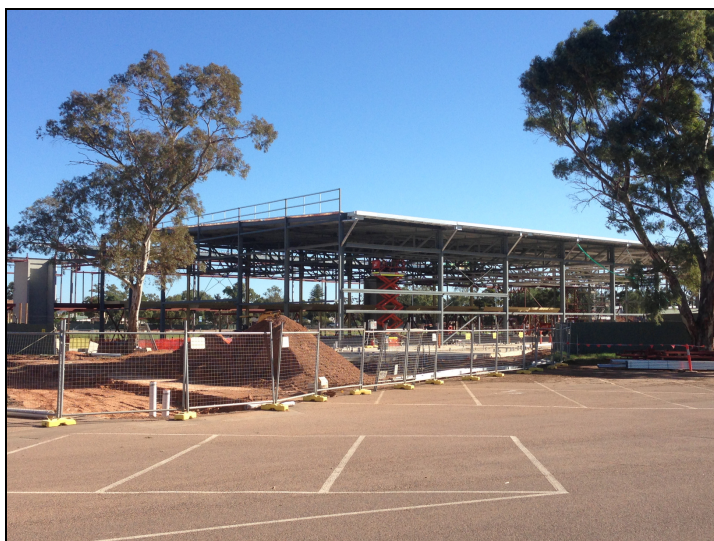
Latest view of the new facility
