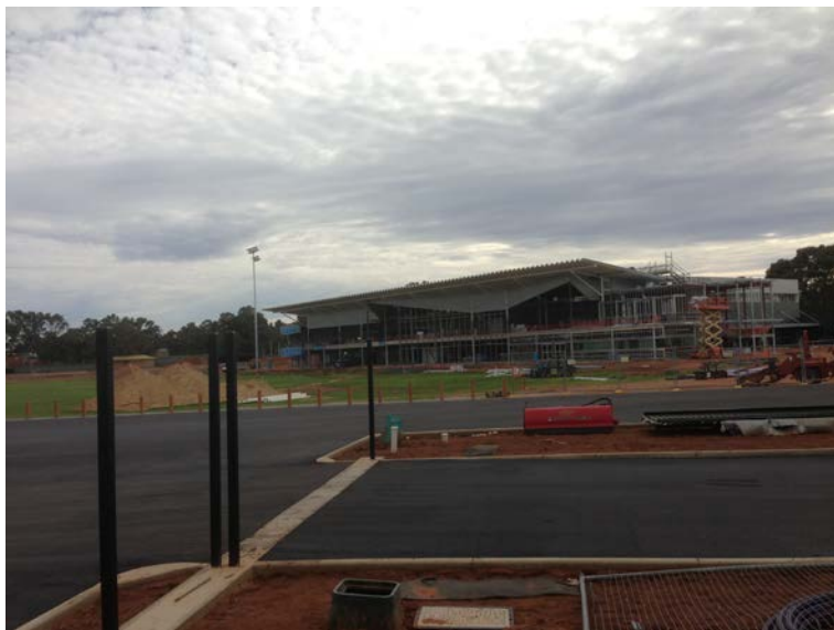
Picture of new complex progress so far
